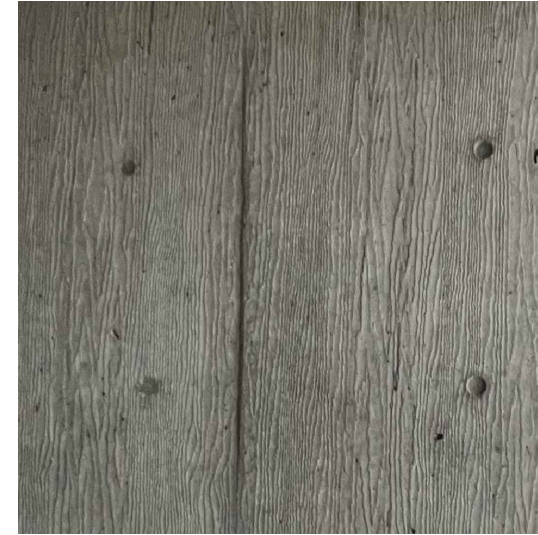
CO1 CONCRETE TO MATCH EXISTING
