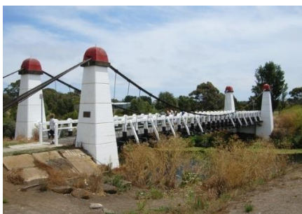
Wollaston Bridge, Warrnambool
