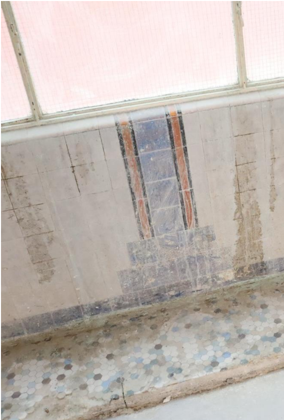
Original tiled sill detailing (outside Mecca tenancy)
