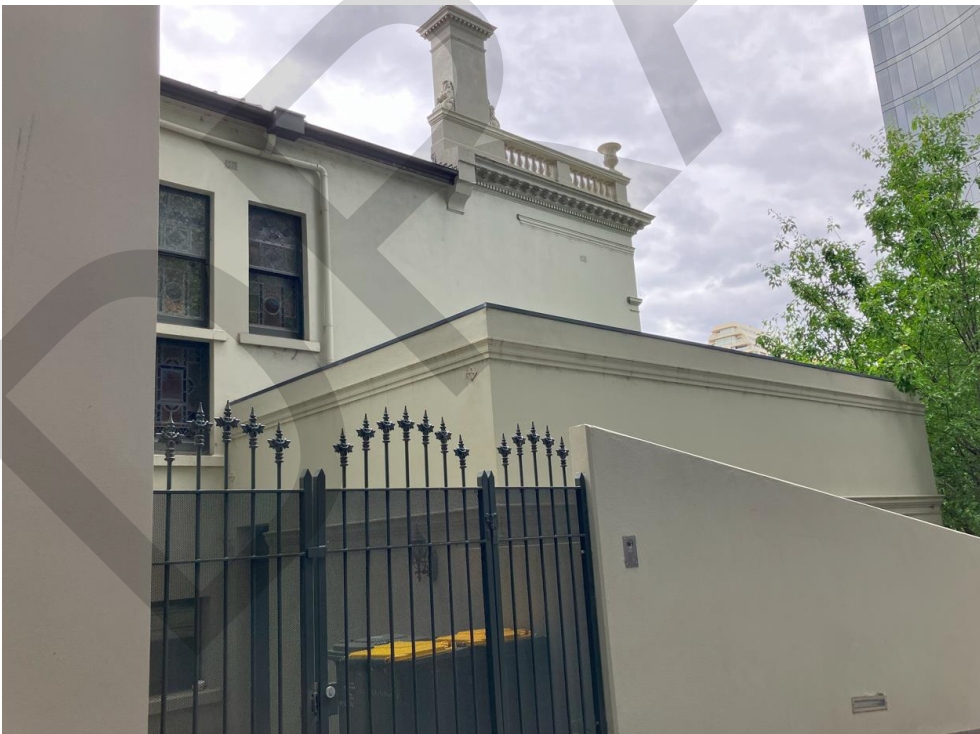
Figure 9 View to the rear of the modified single-storey rear component of the building; the leadlight windows on the rear elevation are visible in this image
