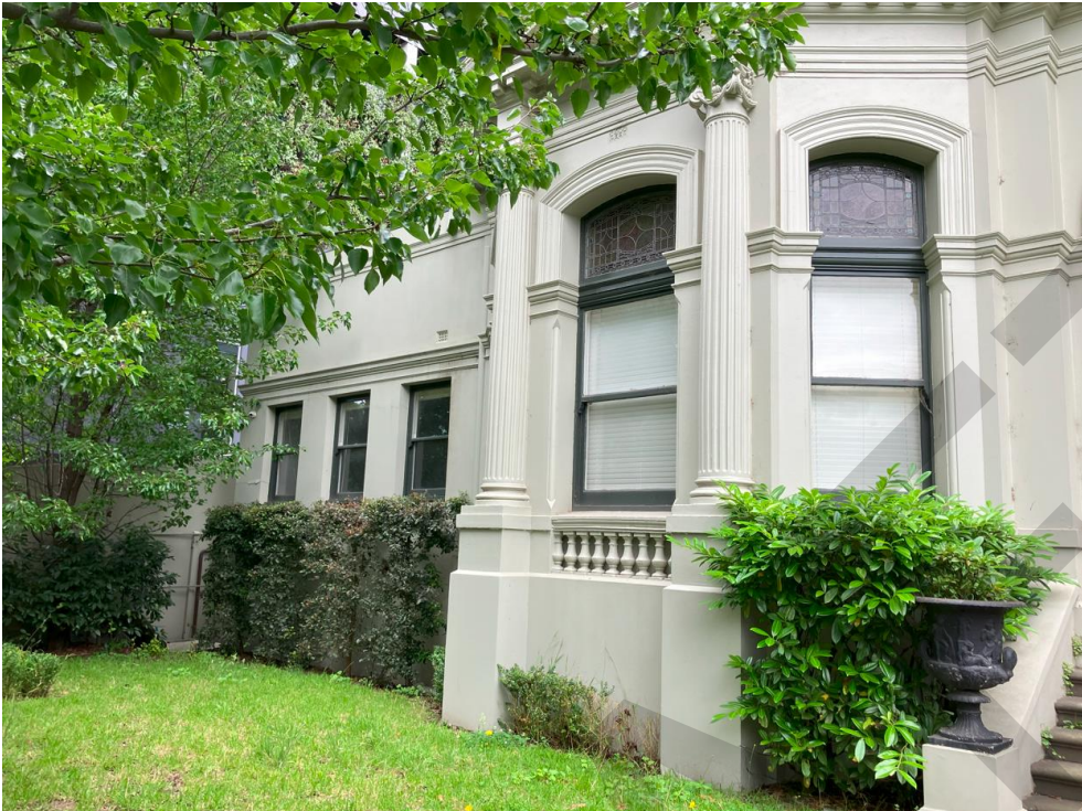
Figure 8 View to the rear of the south elevation showing the 1930s addition to the original building
