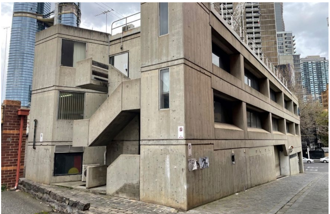
Figure 10 Rear (north) and west elevations
