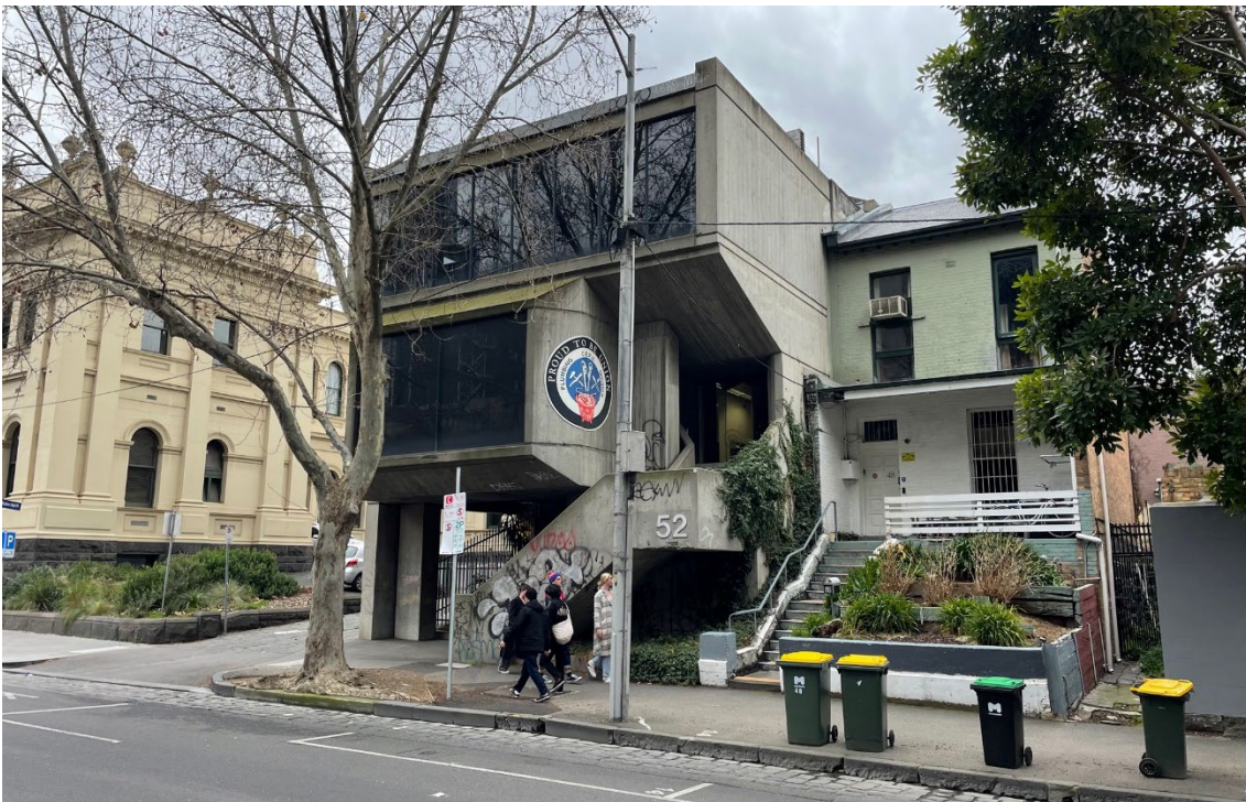
Figure 8 South elevation, looking north-west from Victoria Street
