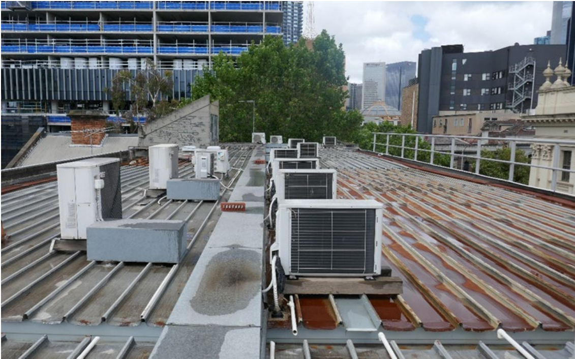
Figure 11 View of the roof, looking south
