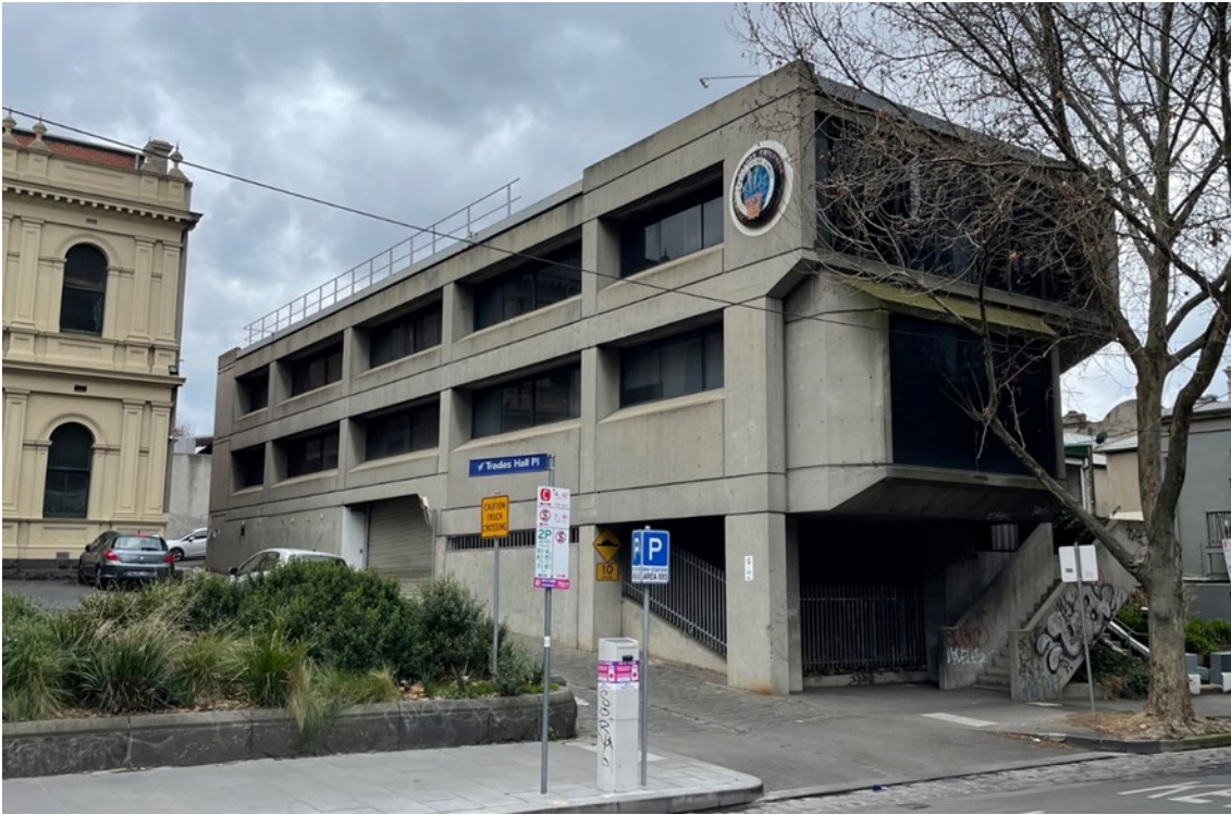
Figure 7 West and south elevations: view from Victoria Street
