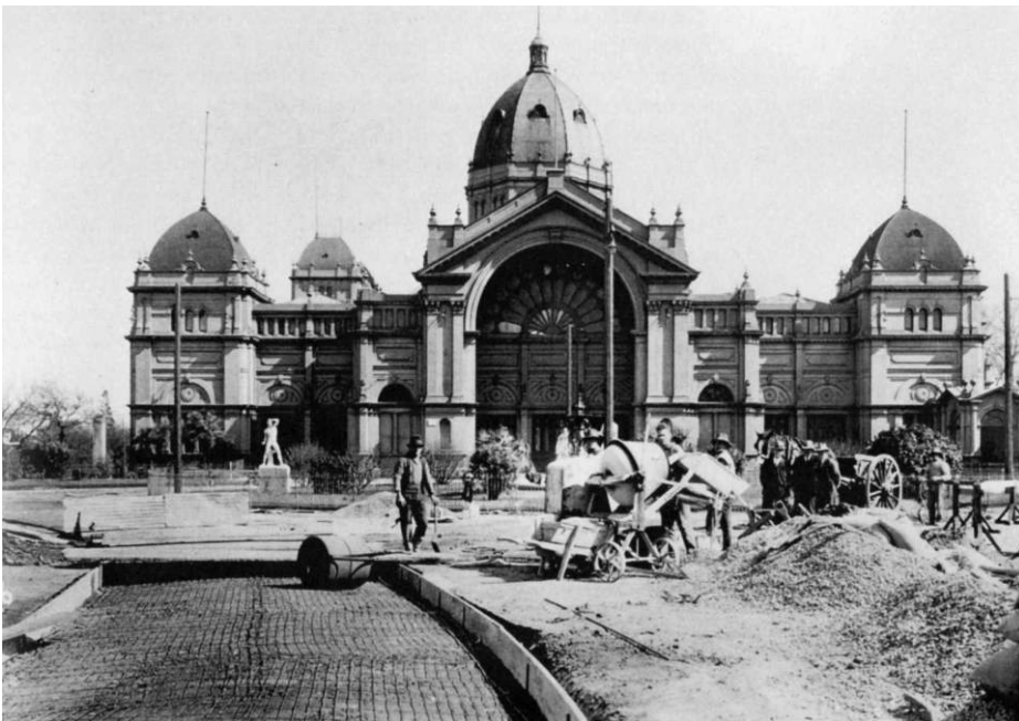
Figure 71 Pouring concrete for the Nicholson Street entrance driveway at the Exhibition Building in the 1920s. Note that the French Fountain and statuary dating from the Great Exhibitions are still clearly visible. Source: Reproduced from Victorian Icon: The Royal Exhibition Building Melbourne .
