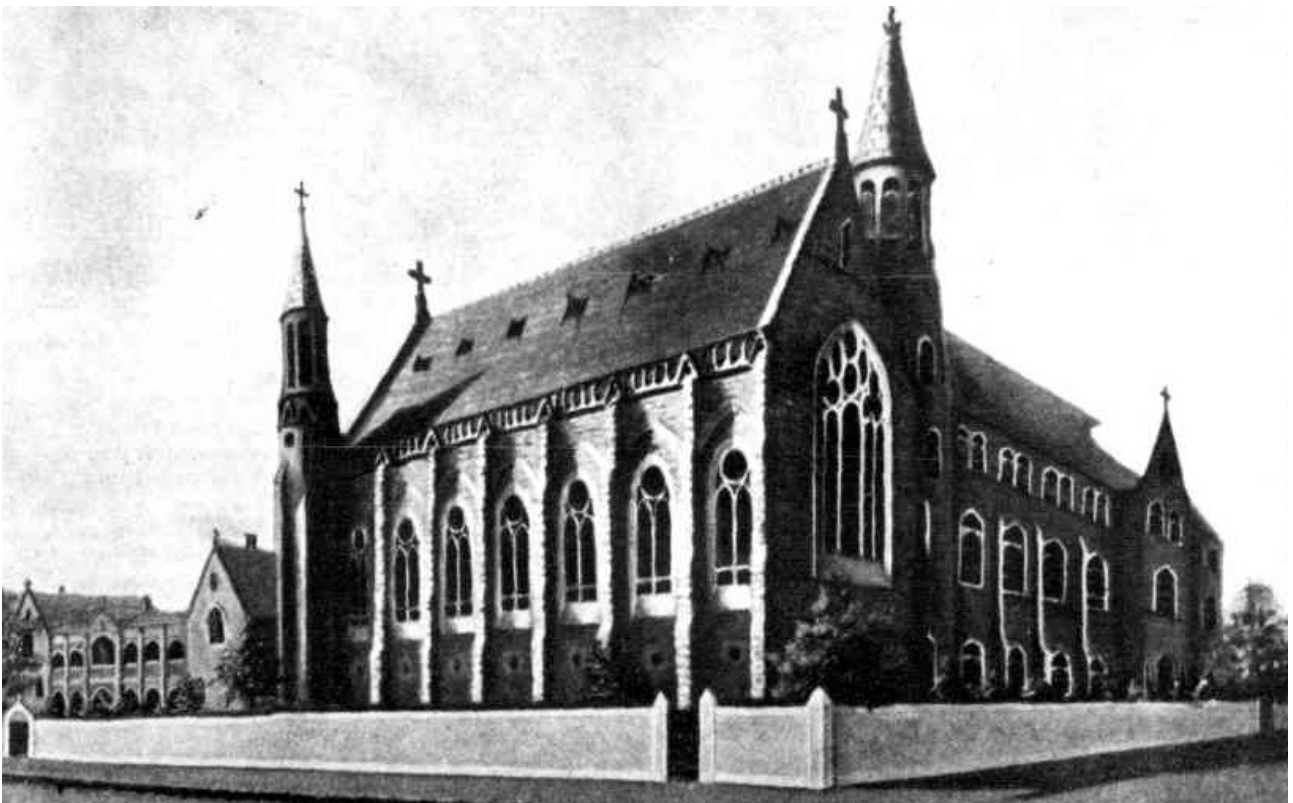
Figure 25 Academy of Mary Immaculate's new high brick fence illustrating the consolidation of the complex Source: 'Convent of Mary Immaculate', Advocate , 31 August 1933
