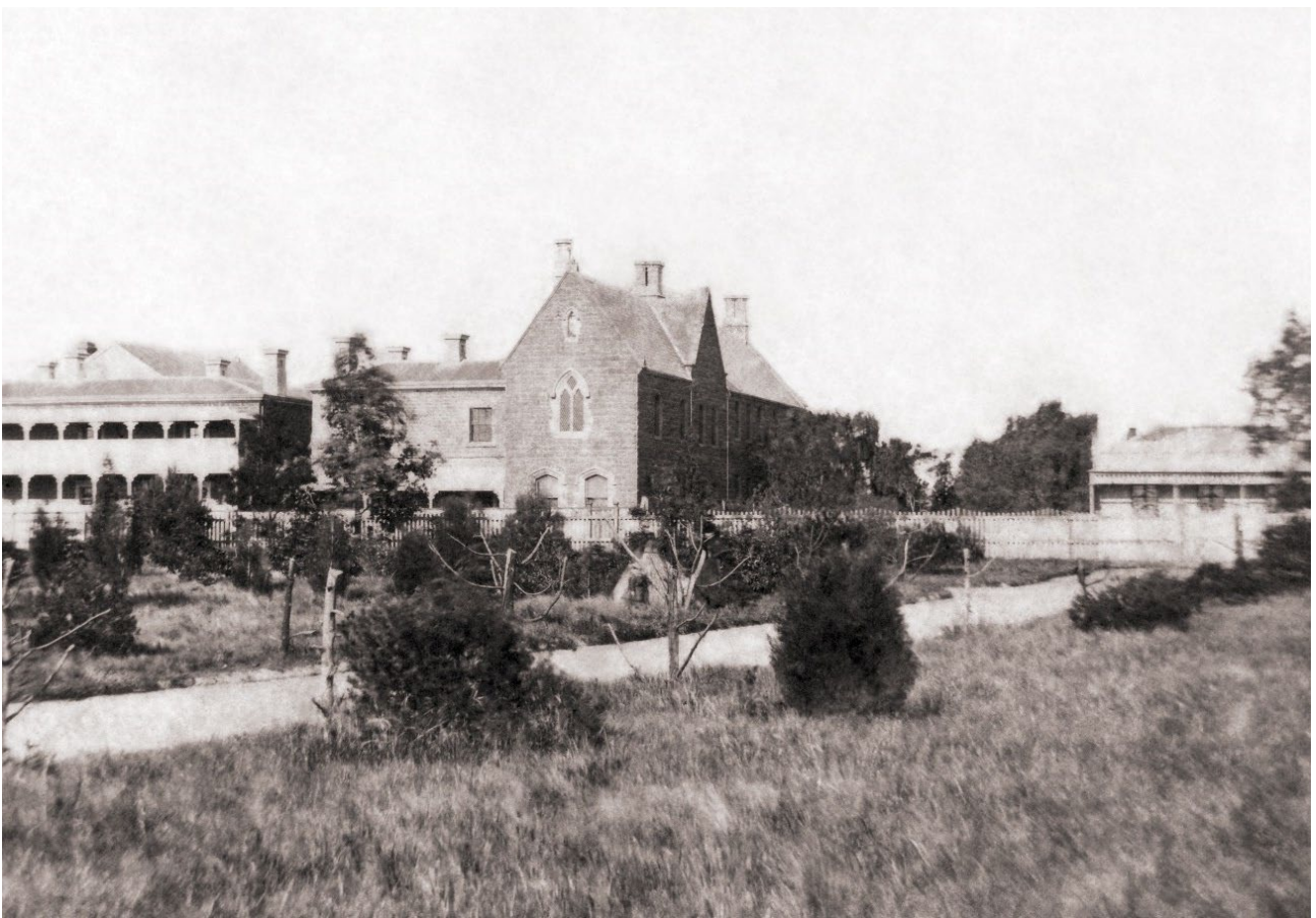
Figure 6 View of the Sisters of Mercy school and convent buildings following 1860s additions Source: Academy of Mary Immaculate archives
