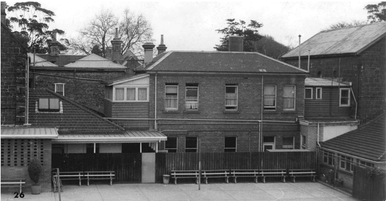
Figure 21 East elevation of the convent showing the various c. 1920s and 1930s weatherboard infills in between the Twelve Sisters House and Kennedy's Residence Source: Kenneth Ko & Frank Wu, History Thesis of the Convent of Mercy Nicholson Street, Fitzroy, 1968
