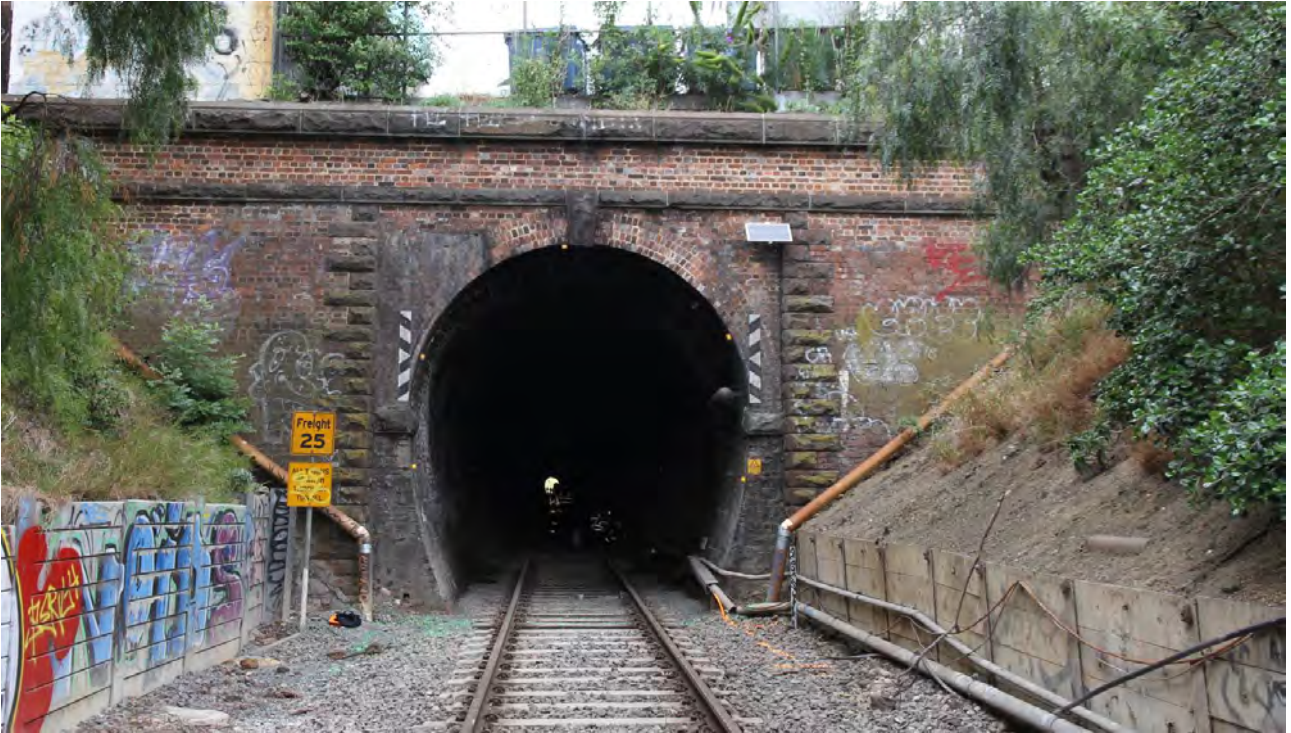
FIGURE 7: VIEW OF UP-END PORTAL OF GEELONG RAILWAY TUNNEL. (SOURCE: ACG)
