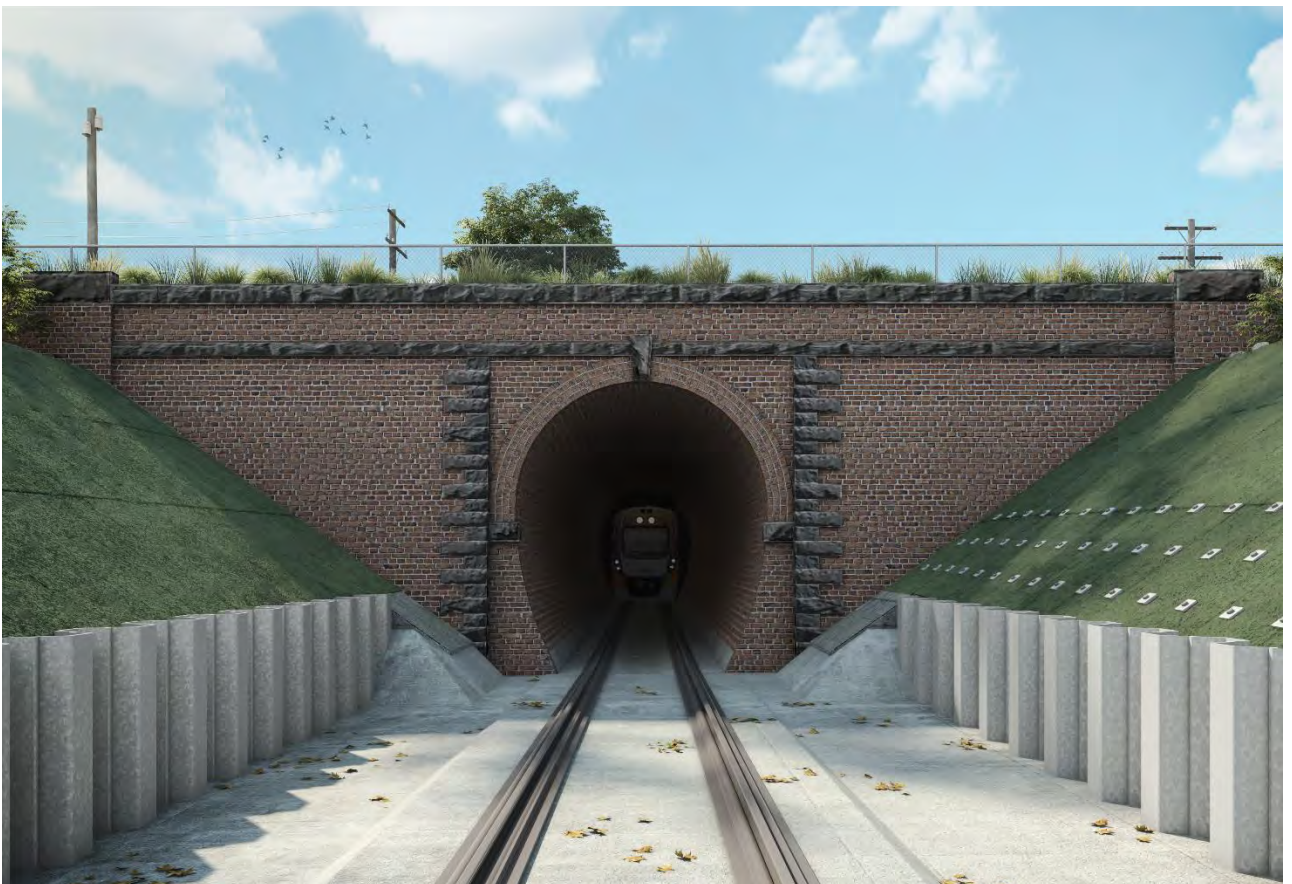
FIGURE 28: 3D VISUALISATION SHOWING THE DOWN-END PORTAL AFTER COMPLETION OF RETAINING WORKS (SOURCE: ACG IMAGE)
