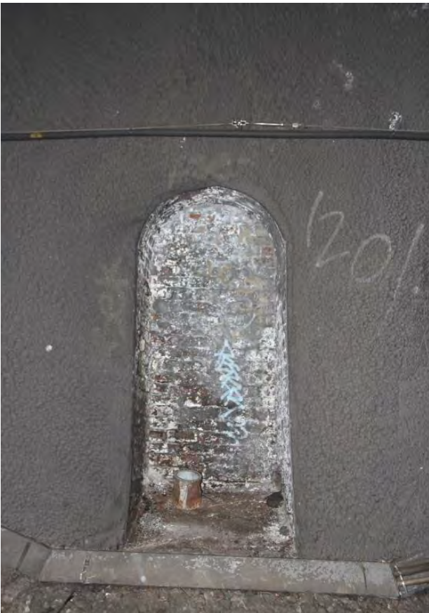
FIGURE 16: INTERNAL VIEWS SHOWING CONDITION OF REFUGES. (SOURCE: ACG)
