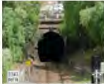
RAILWAY TUNNEL SOHE 2008
