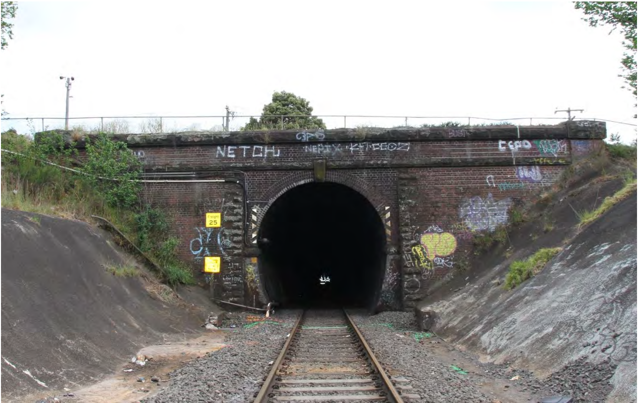
FIGURE 27: EXISTING VIEW OF DOWN END PORTAL (SOURCE: ACG)
