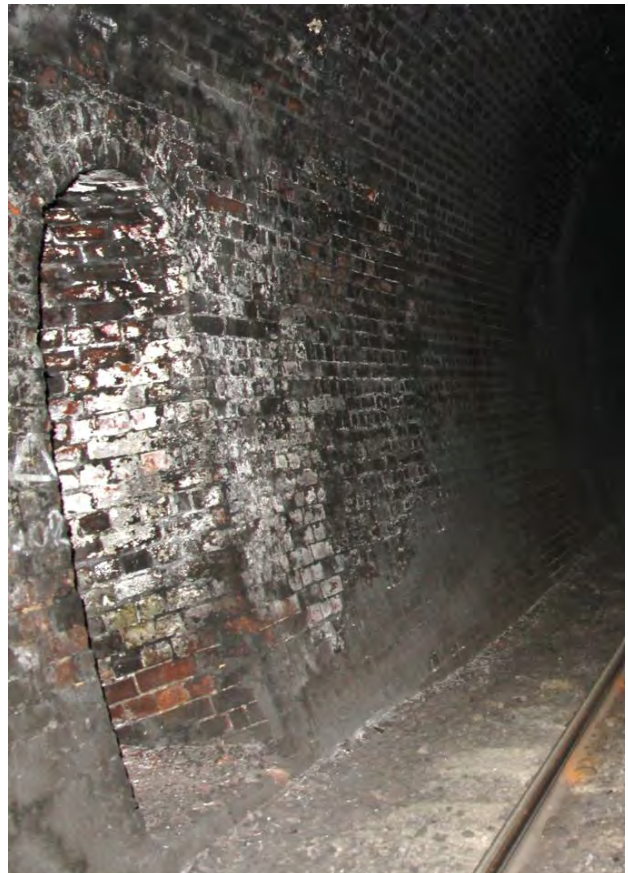
FIGURE 15: INTERNAL VIEW OF TUNNEL SHOWING CONDITION OF BRICK LINING, TRACK AND SERVICES – LOOKING SOUTH. (SOURCE: ACG) NOTE: TUNNEL STRUCTURAL DESIGN REPORT MENTIONED THIS SHOTCRETE ON WALLS AND PUMPING GROUT BEHIND LINING TO FILL VOIDS WAS DONE IN 1995.
