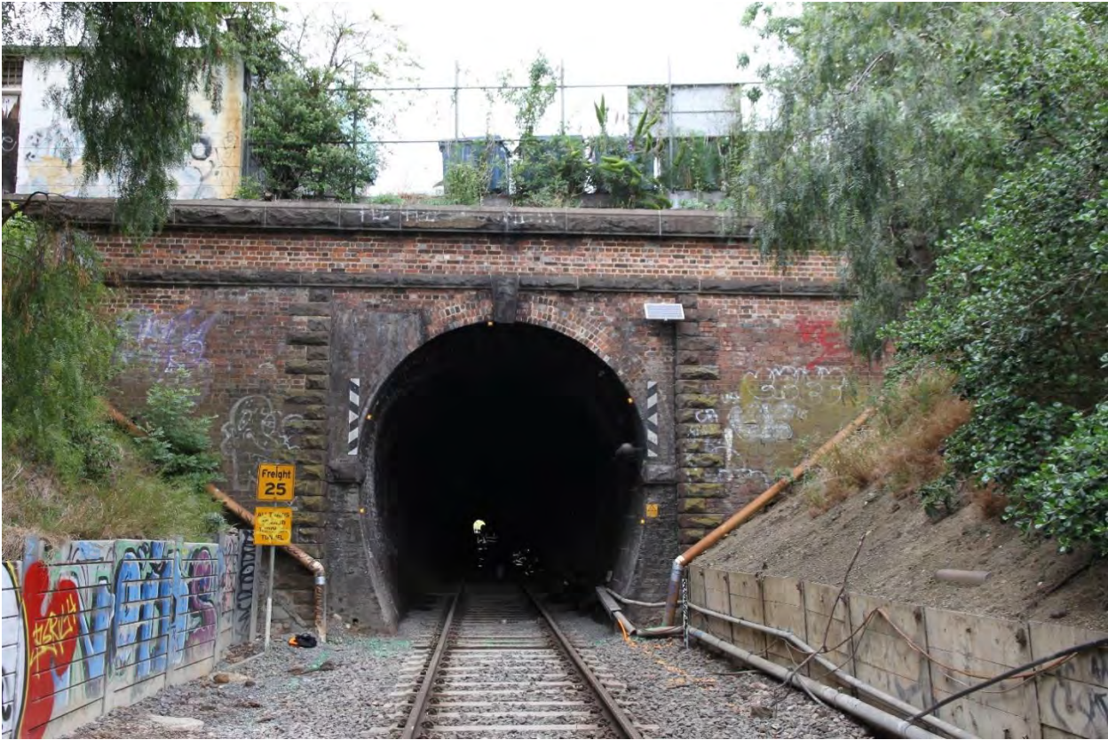
FIGURE 37: EXISTING UP END PORTAL (SOURCE: ACG IMAGE)
