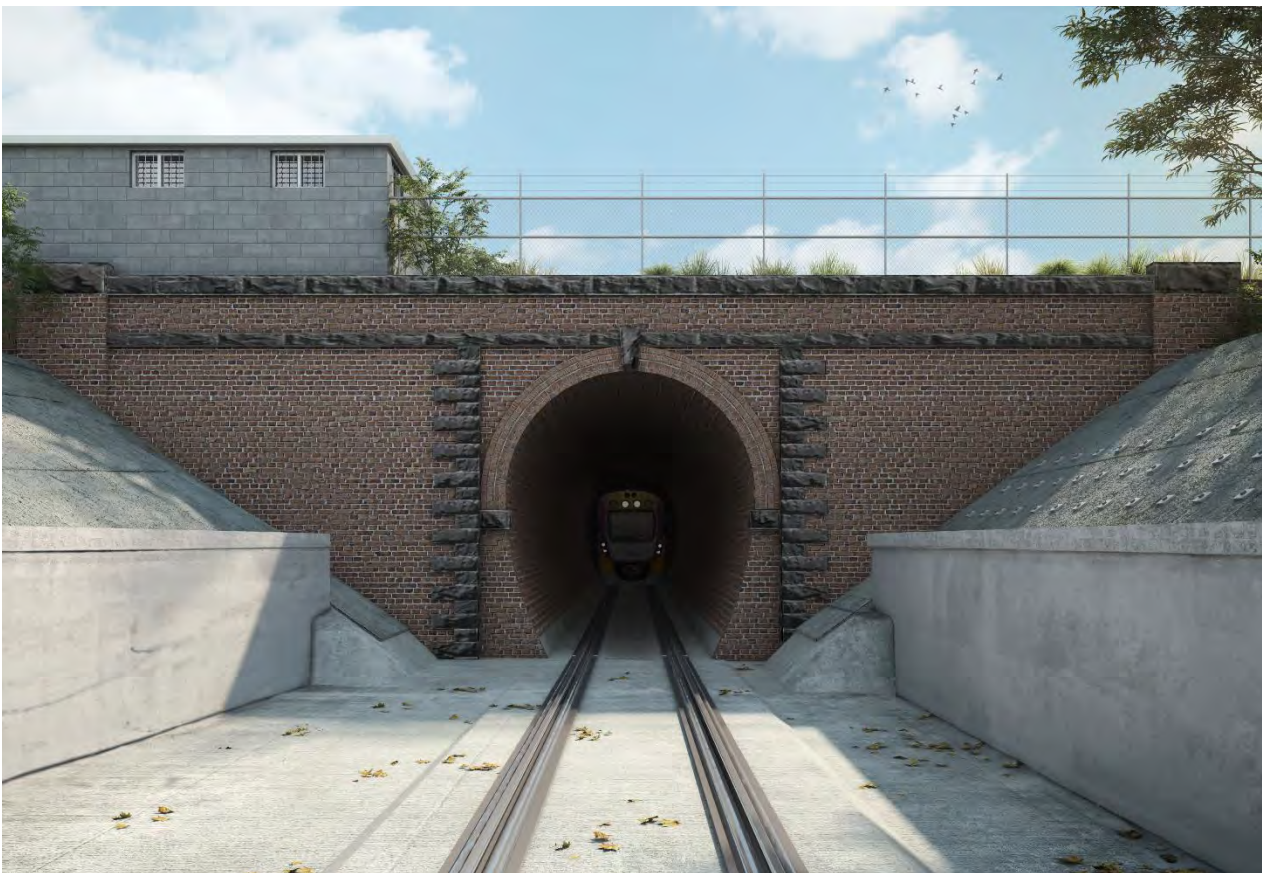
FIGURE 38: 3D VISUALISATION SHOWING THE UP-END PORTAL AFTER COMPLETION OF RETAINING WORKS
