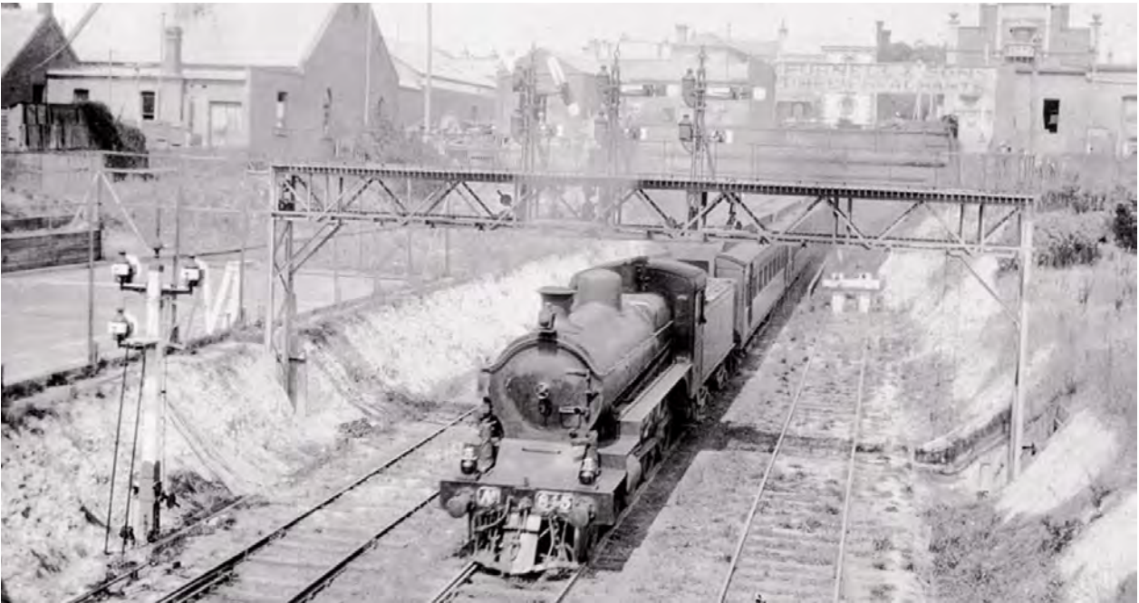
FIGURE 5: CIRCA 1930 PHOTOS SHOWING A2 845 EXITS THE GEELONG TUNNEL ON AN UP PORT FAIRY PASS. (SOURCE: VICTORIANRAILWAYS.NET)
