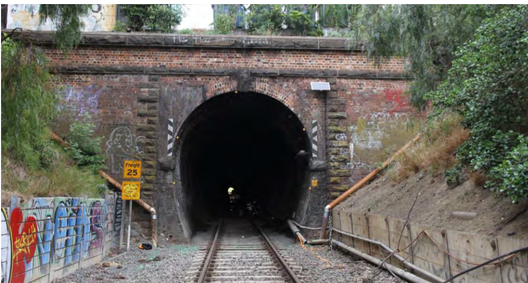
FIGURE 1: VIEW OF UP-END PORTAL OF GEELONG RAILWAY TUNNEL (SOURCE: ACG 2023)
