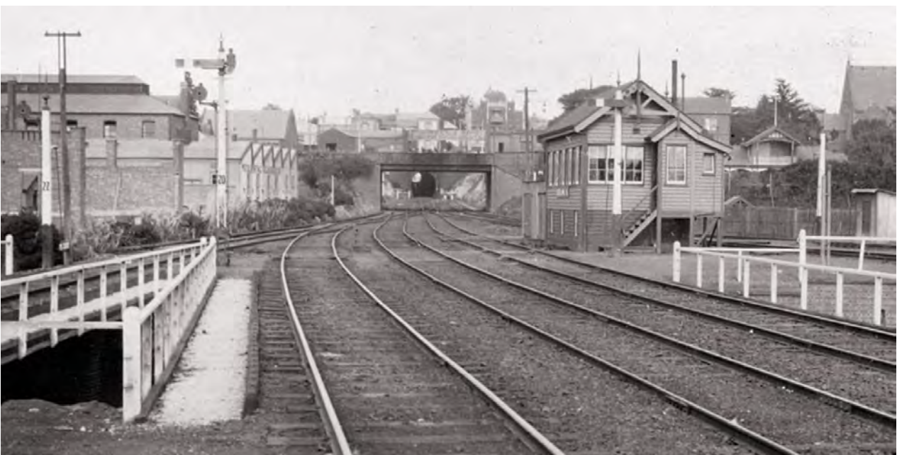
FIGURE 6: UNDATED PHOTOS TAKEN FROM THE PLATFORM AT GEELONG LOOKING SOUTH TOWARDS THE TUNNEL. THE SIGNALBOX ON THE RIGHT WAS GEELONG B BOX (SOURCE: VICTORIANRAILWAYS.NET)
