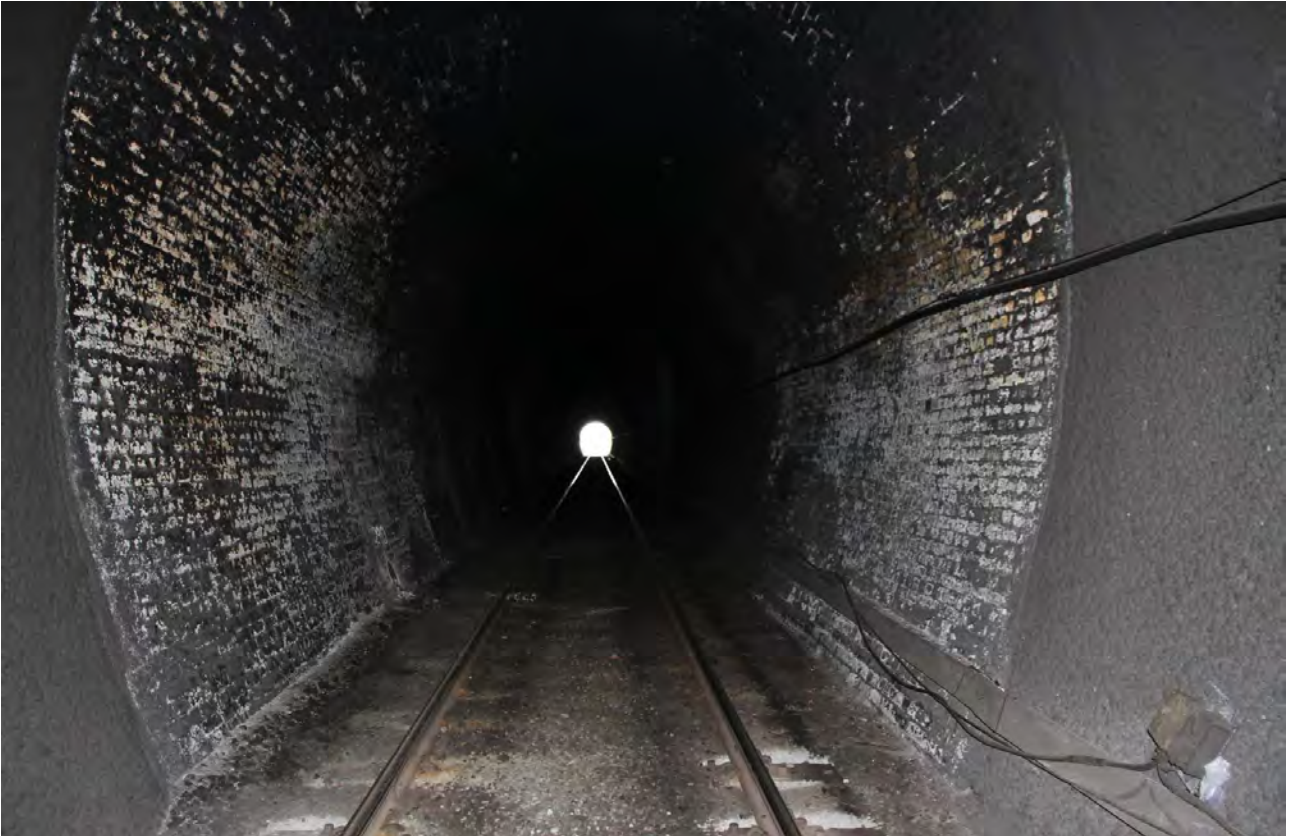
FIGURE 15: INTERNAL VIEW OF TUNNEL SHOWING CONDITION OF BRICK LINING, TRACK AND SERVICES – LOOKING SOUTH. (SOURCE: ACG) NOTE: TUNNEL STRUCTURAL DESIGN REPORT MENTIONED THIS SHOTCRETE ON WALLS AND PUMPING GROUT BEHIND LINING TO FILL VOIDS WAS DONE IN 1995.
