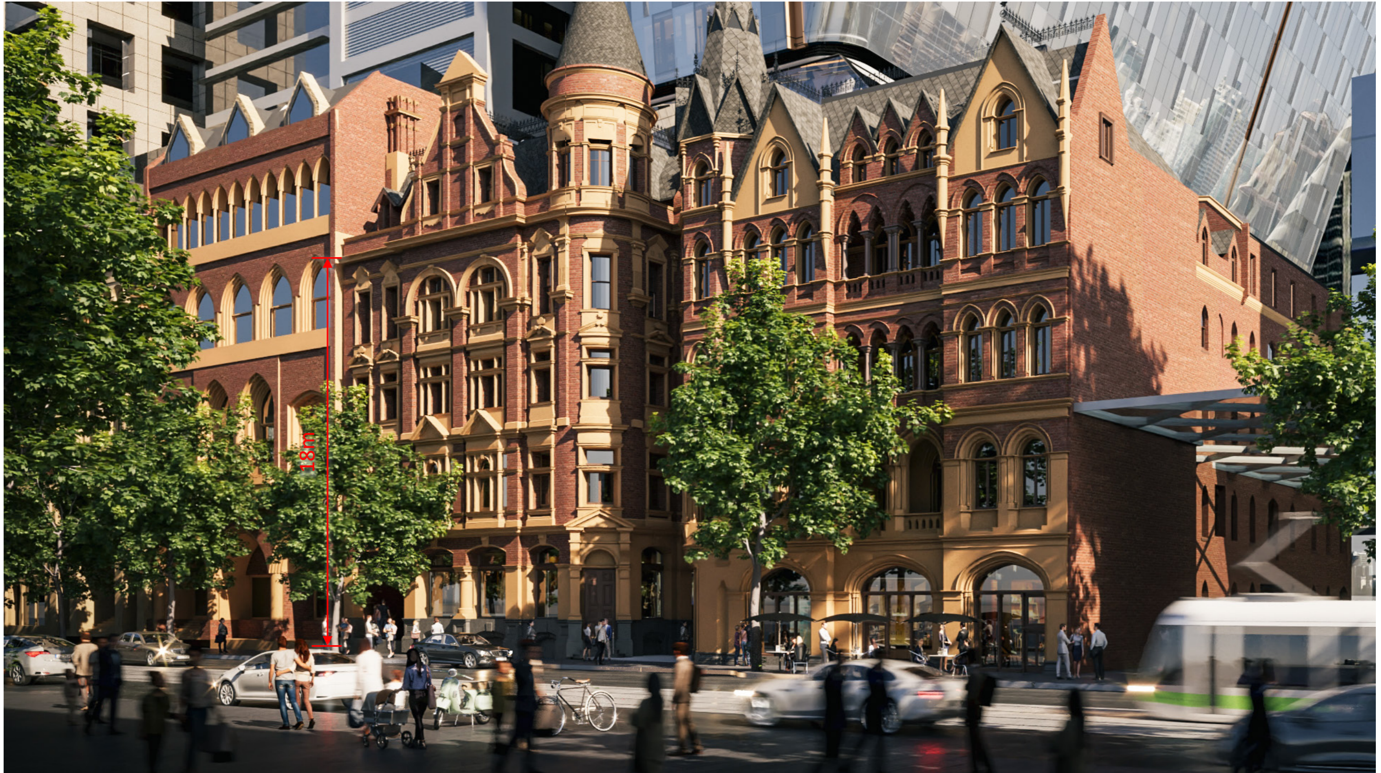
Collins Street level view showing the west façade of the Rialto Building. Dimension showing 18m which is considered the typical field of view for a street level pedestrian.
