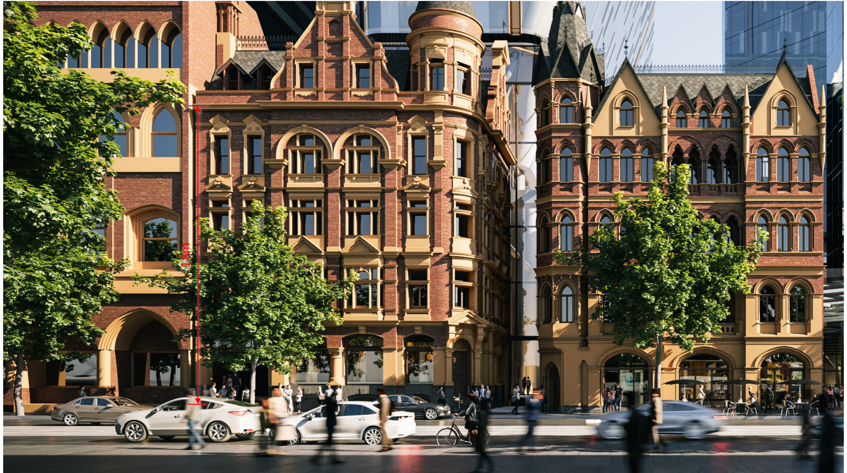
Collins Street level view from directly in front of the Rialto Building. Dimension showing 18m which is considered the typical field of view for a street level pedestrian.
