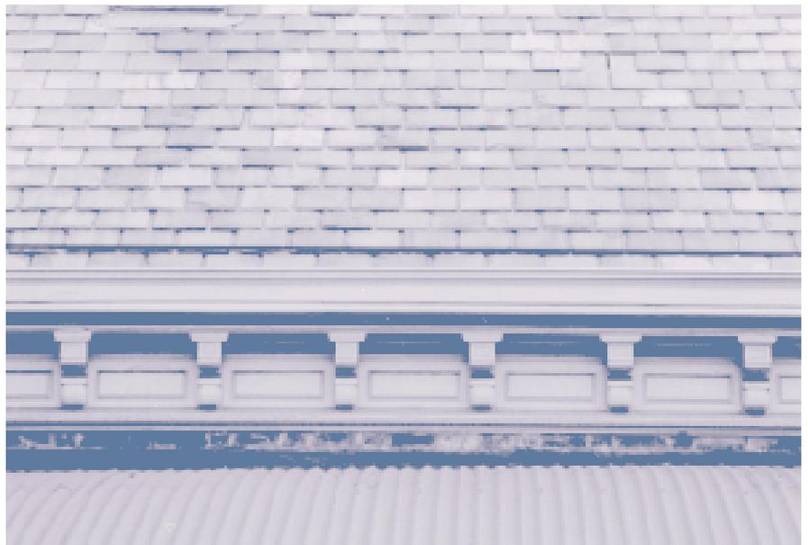
*Spanish slates used to replace Welsh slates show bleeding of ferrous oxides and some delamination only 10 years after placement on this railway station roof.*
