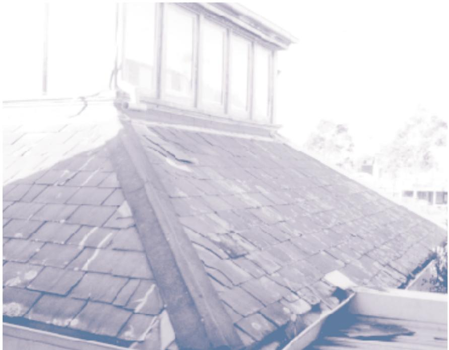
*Slipping slates in the worst possible location: directly below a rainwater spreader.*
