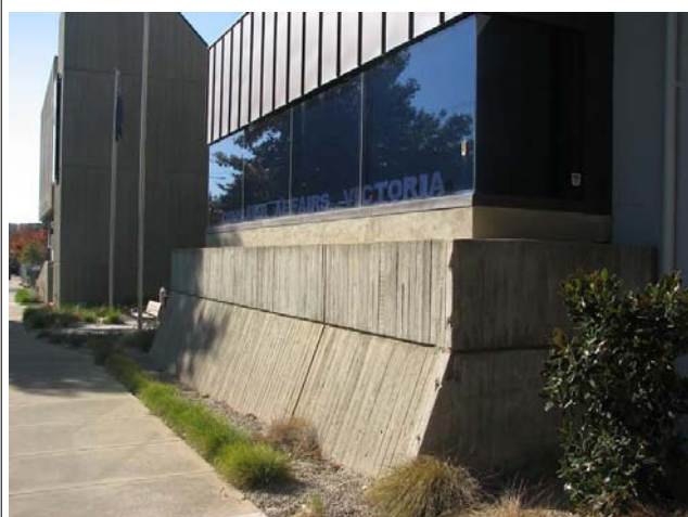
Detail of Ovens Street (west) frontage, showing battered base
