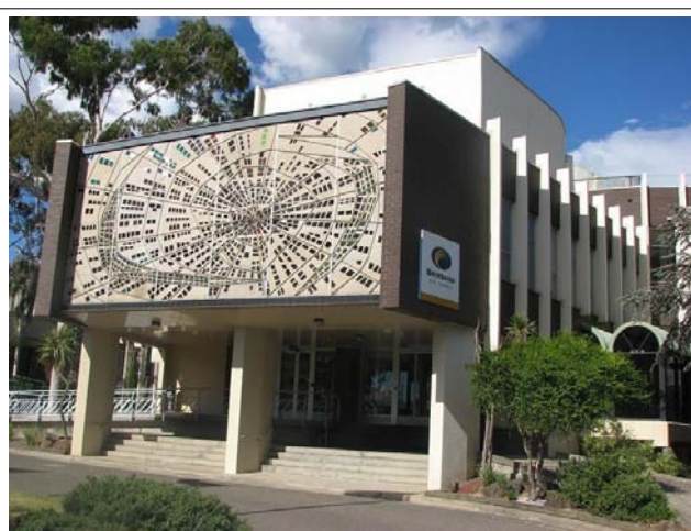
Main entry portico, with dalle de verre window at upper level
