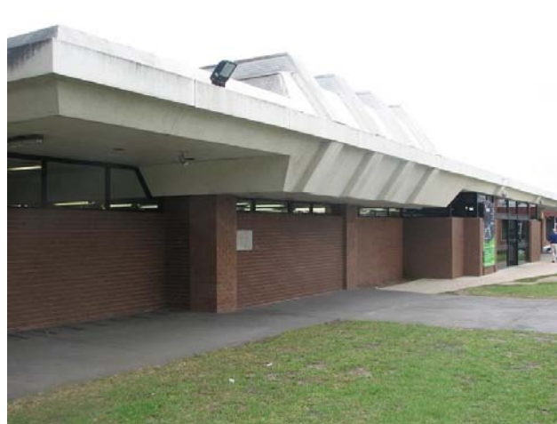
Rear facade, showing stepped roofline and bricked-up entrance
