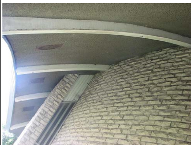
Underside of dome, showing ribs and rendered finish
