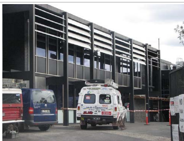
North side of original 1966-67 building; note fixed louvres
