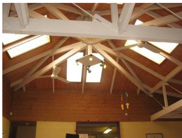
Detail of interior showing exposed roof truss
