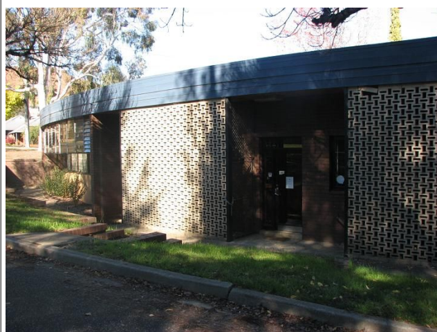
Rear of office block, showing screen walls and glass louvres
