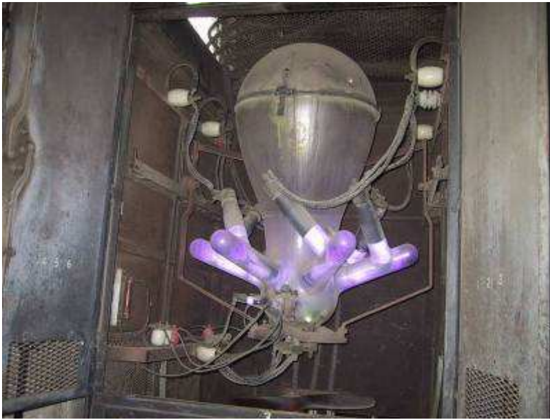
Figure 123: Mercury Arch rectifier in Preston Substation (photo Robert Green)
