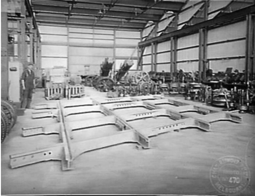
Figure 108: Tram track crossover fabricated at Chas Ruwolt Pty Ltd, Richmond, Museum Victoria image MM 011937
