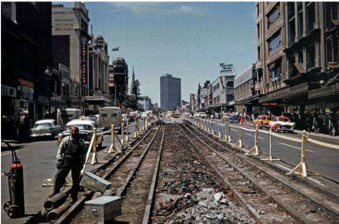
Figure 16: Cable tram tracks being removed from Lonsdale Street in February 1962. 66
