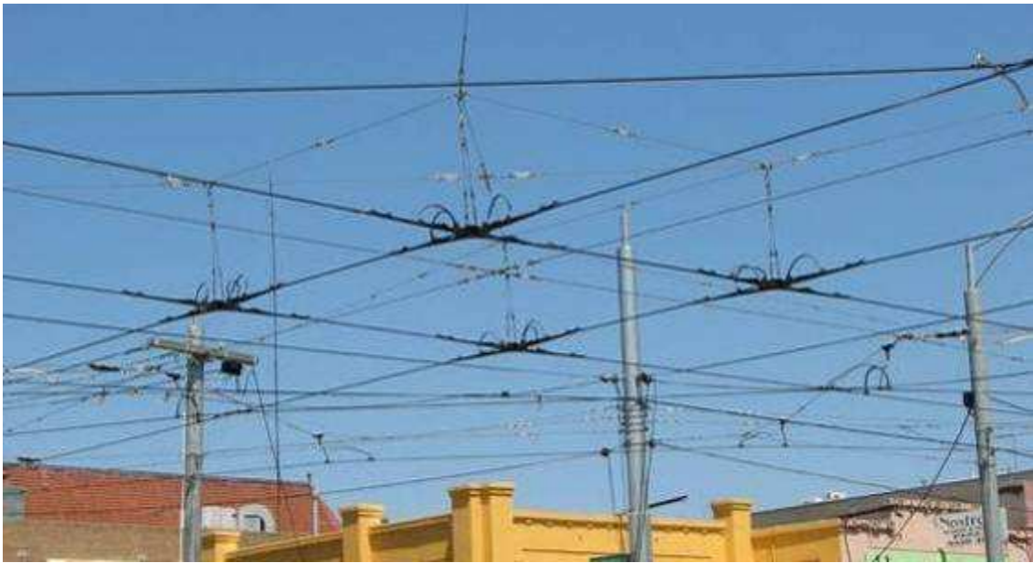
Figure 106: Overhead wires at Grand Union Junction, Balaclava after it was rewired to get rid of frog pans.
