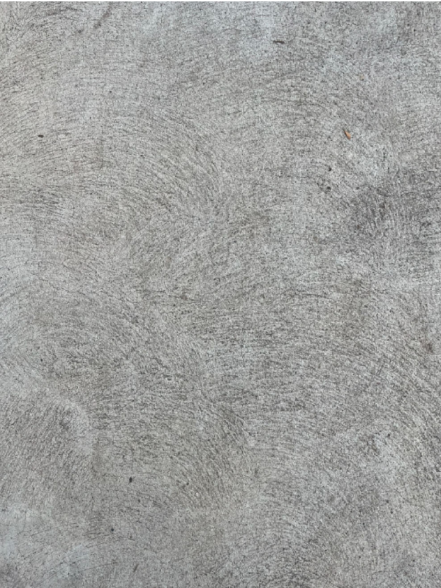
CONCRETE STEPS / SEAT / PODIUM - formed concrete with float finish, recycled aggregate
