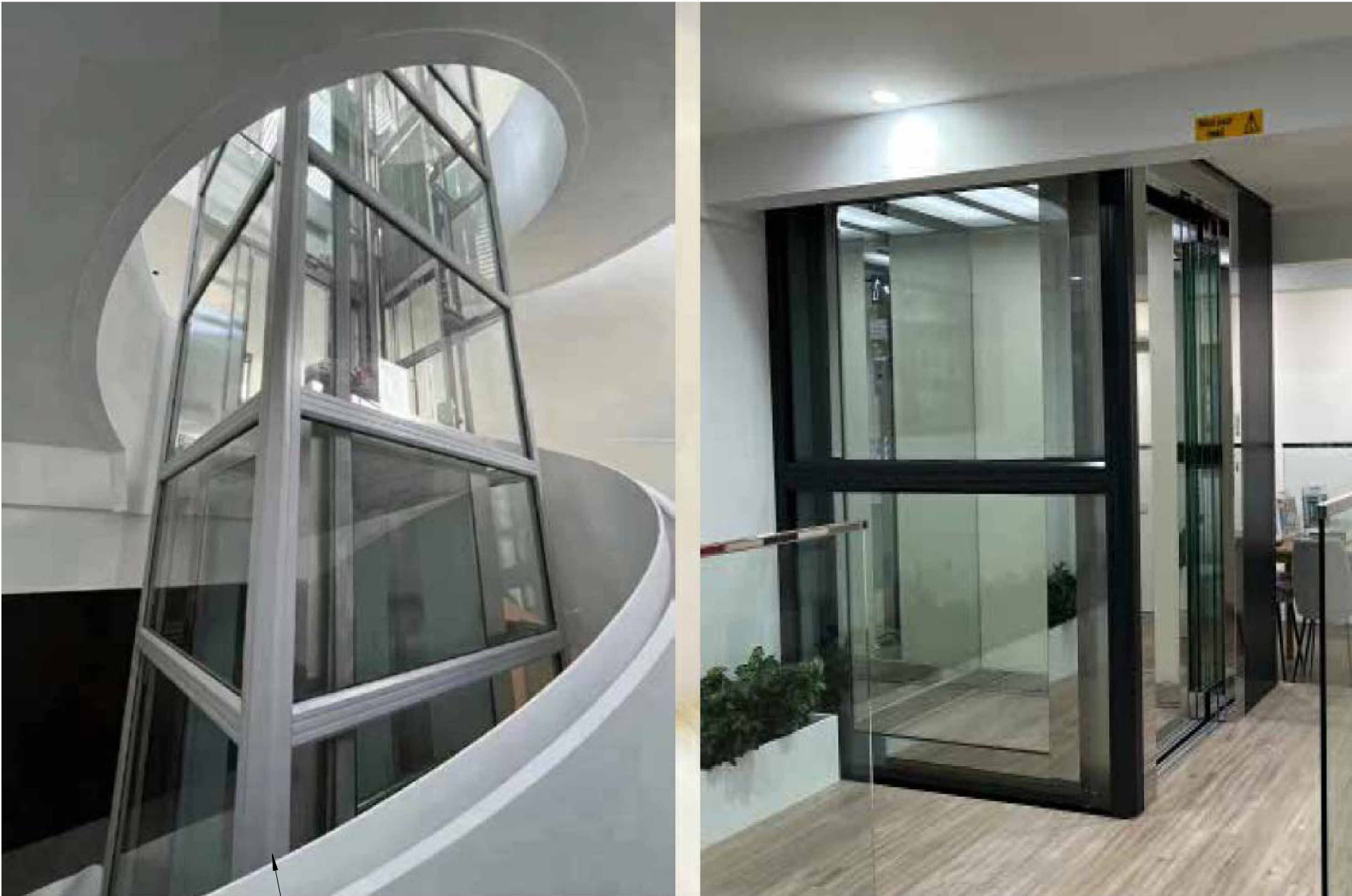
Ecotrack series 3 or equivalent elevator with full glazed lift shaft to be utilised so original building fabric is on display
