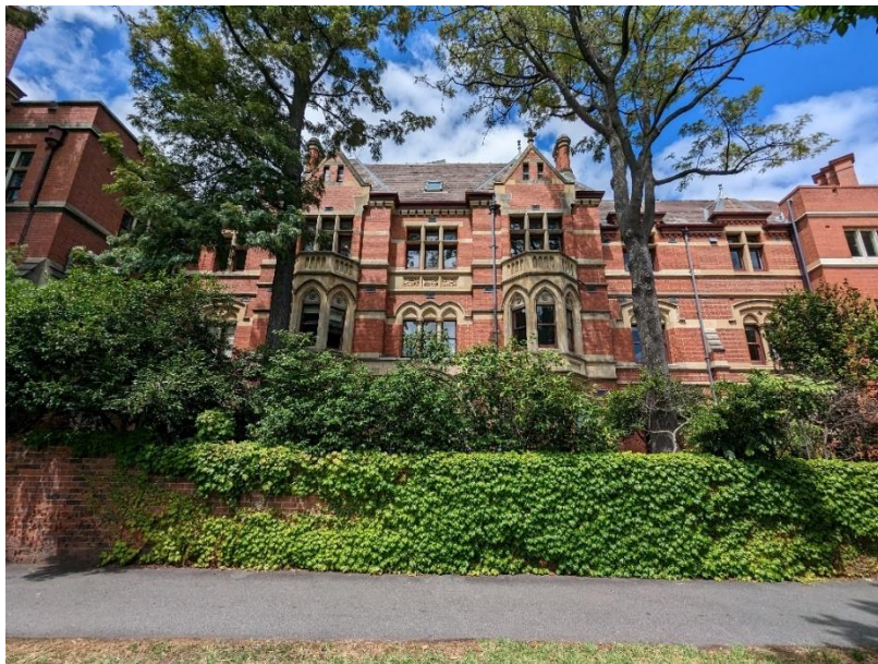
Figure 2, Janet Clarke Hall principal facade addressing College Crescent (February 2023)
