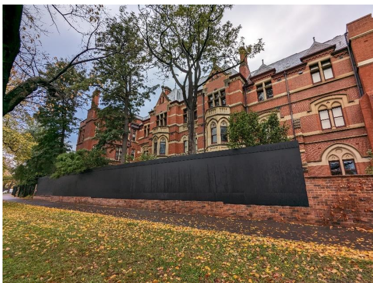
Figure 5, Partially demolished fence following permit exemption works (June 2023)
