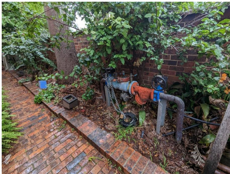
Figure 4, existing condition of the courtyard behind the wall/fence (2023)
