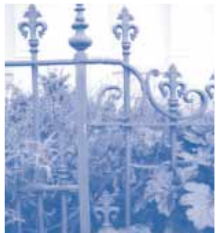
This residential scale palisade style fence is made of wrought iron and cast iron components.
