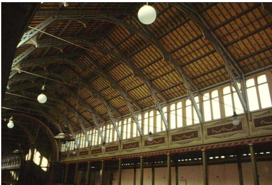
Figure 52 Detail of roof framing and clerestory in nave.
