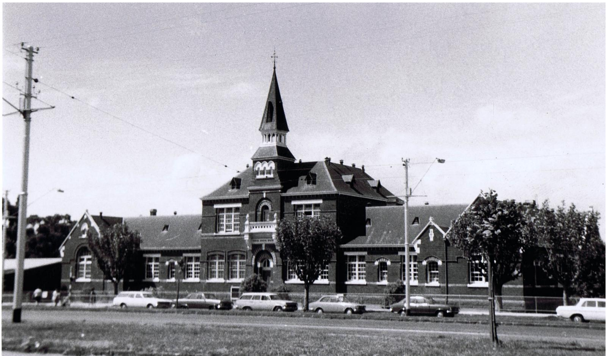
Figure 1," Main school building"/1875 Building with 1878 additions, St Kilda Primary School, Photograph 1971, (Source St Kilda Historical Society/Flicker online)
