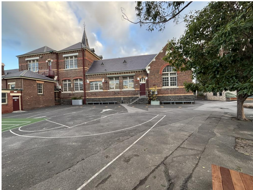
Figure 7, St Kilda Primary School, rear facade and grounds showing proposed landscape development area, Photograph 2025
