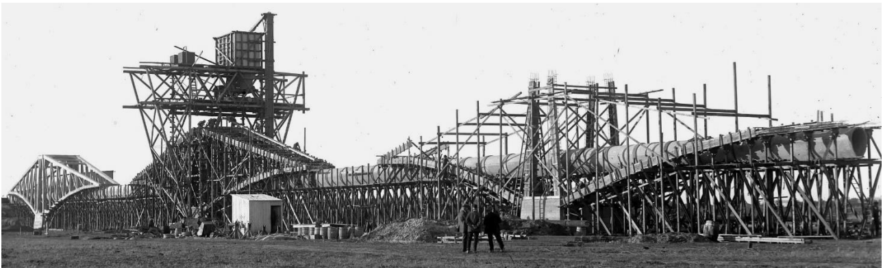
Figure 13 Construction sequence (c.1914) with (right) temporary scaffolding and timber formwork; (centre left) completed truss formwork and concreting gantry; (far left) complete (but uncapped) concrete web truss Source: Barwon Water archives
