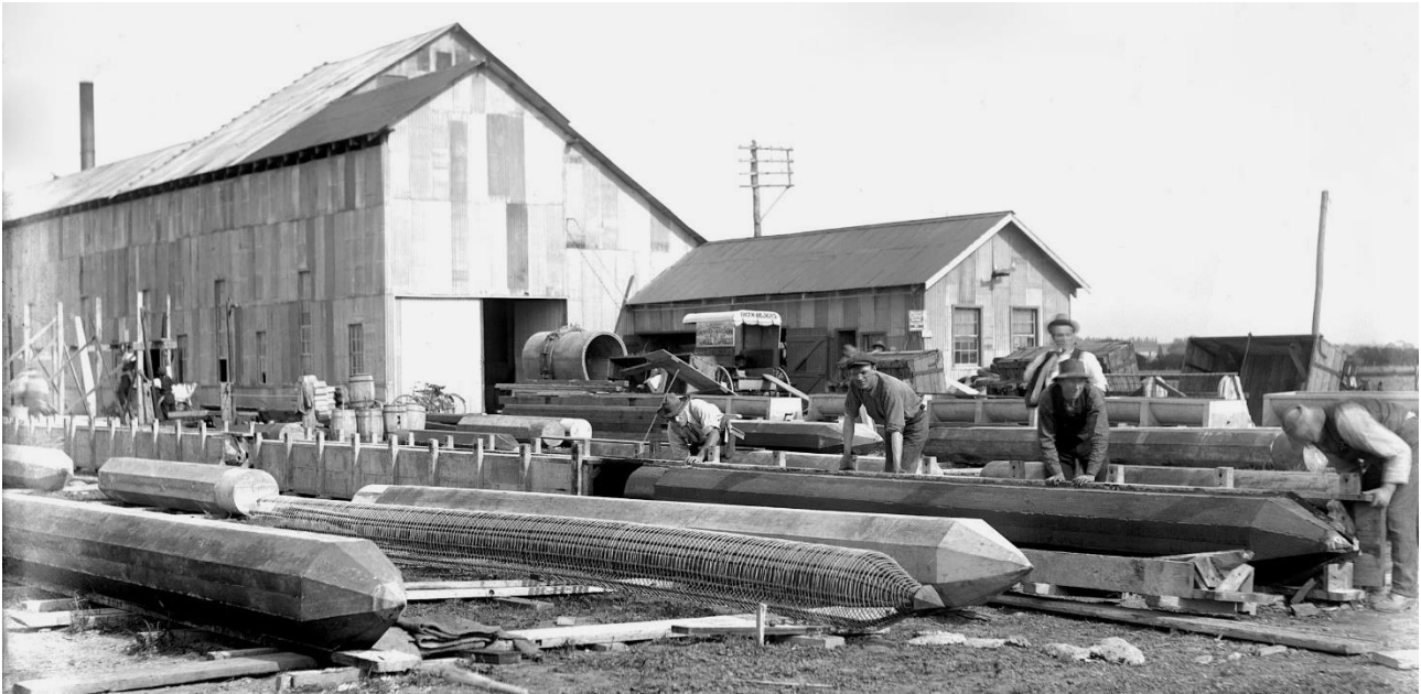
Figure 12 Manufacturing of Aqueduct's precast concrete piles at Stone & Siddeley's Marshall Pipe Factory, 1913 Source: Barwon Water archives
