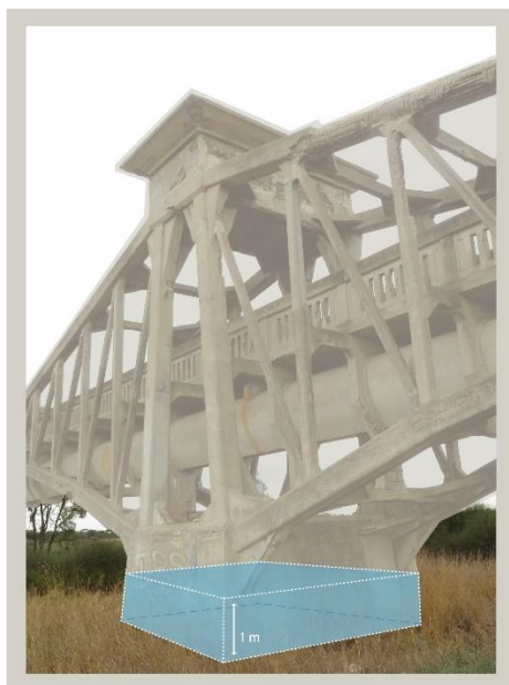
Retention of Pier Bases
