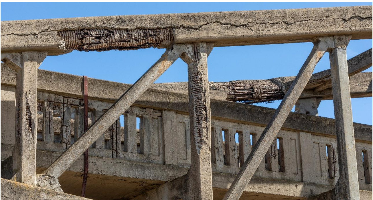
Figure 7 Severe deterioration of two upper truss chords; this type of failure is likely to trigger a sudden collapse Source: Glasshouse Creative Media, courtesy Barwon Water
