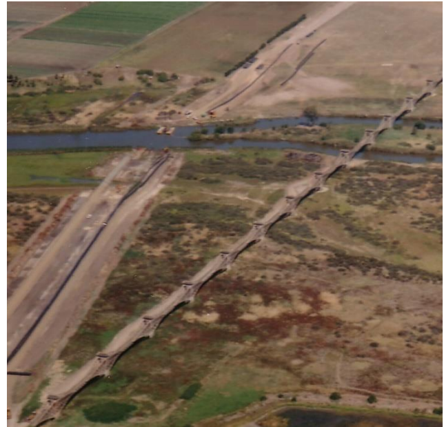
Figure 21 Replacement siphon under construction below Barwon River, c. 1991 Source: Barwon Water archives
