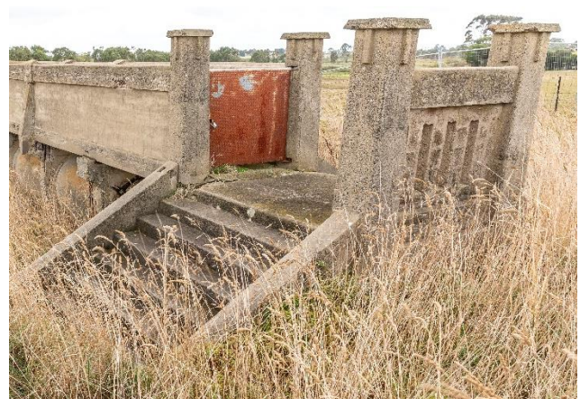
Figure 51 (left) Pier Base 13 (right) South Landing Stair, exposed crown of in-ground ovoid sewer pipe visible in foreground (2019) Source: Lovell Chen archives and Glasshouse Creative Media courtesy Barwon Water
