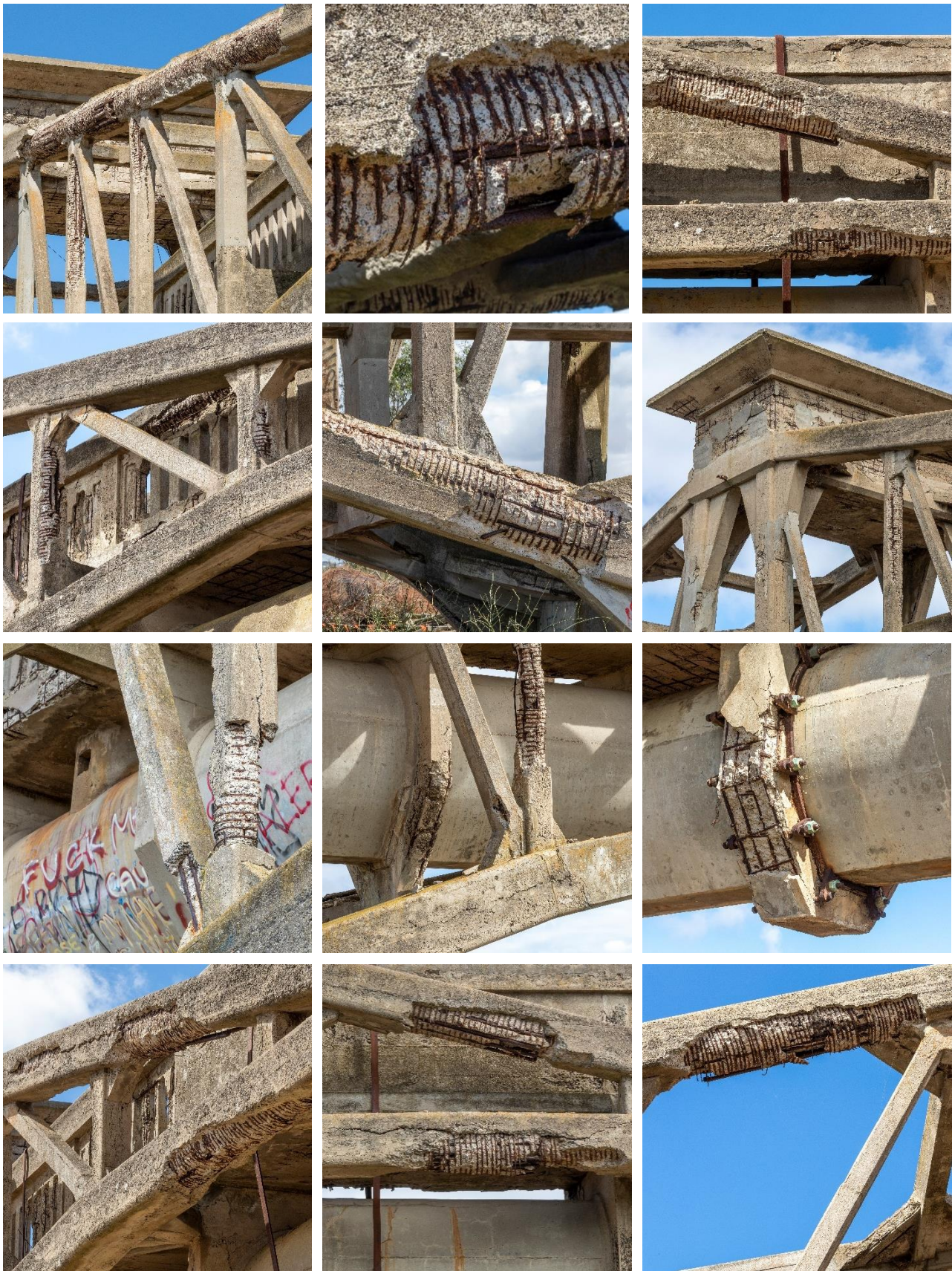
Figure 23 Exemplar deterioration of the concrete cover and underlying steel reinforcement across the Aqueduct Source: Glasshouse Creative Media (2022), courtesy Barwon Water
