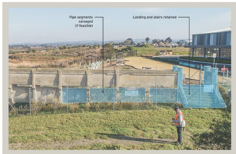
Sewer Landings retained at north and south ends of structure
