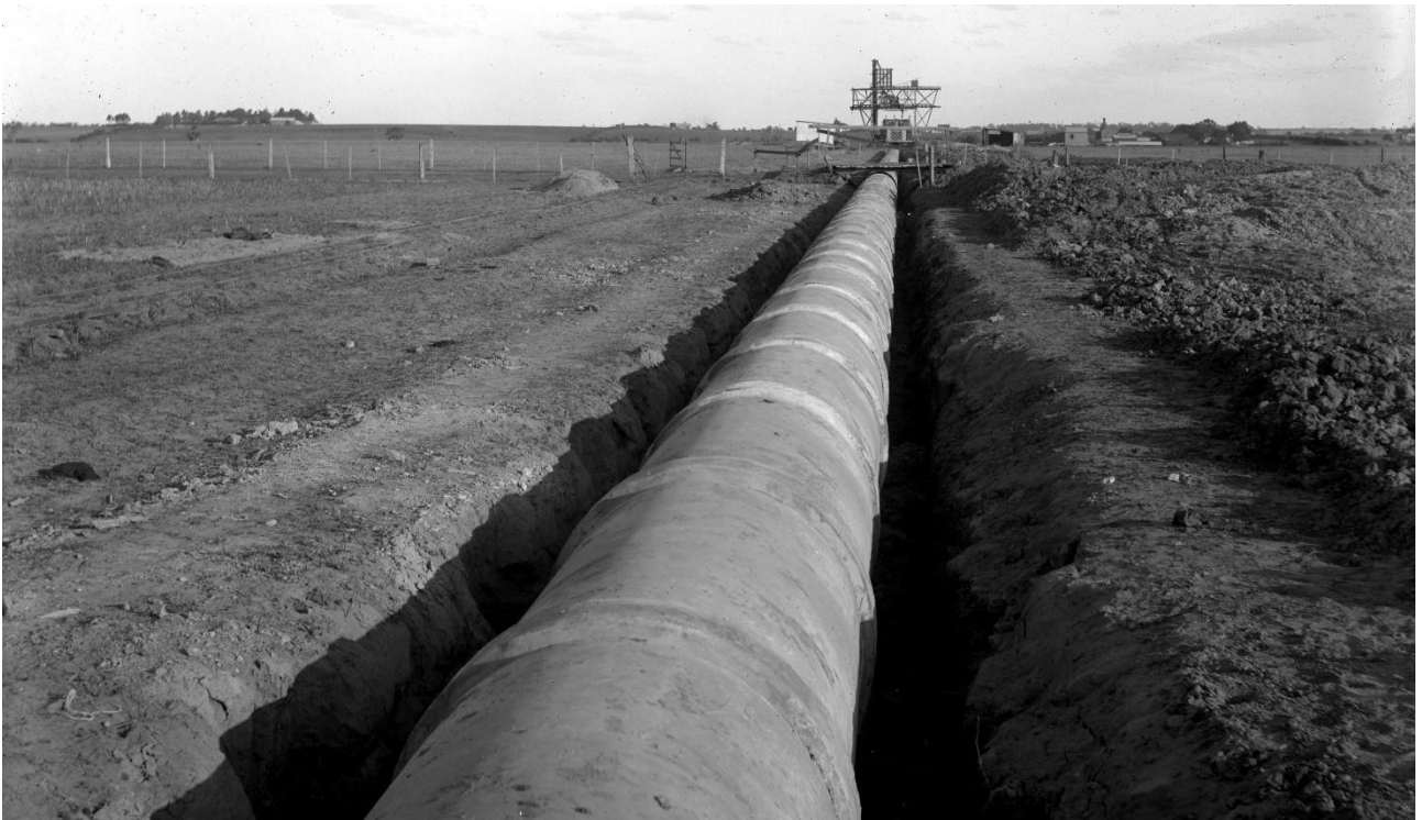
Figure 11 Geelong Outfall Sewer being laid in trench south of Breakwater, 1914 Source: Barwon Water archives
