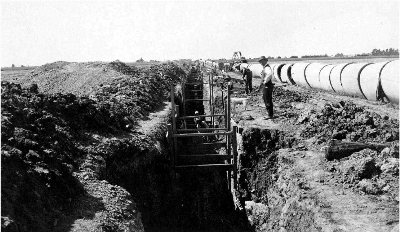
Figure 10 Trenching for installation of the Geelong Outfall Sewer, c. 1912-1914, with ovoid sewer pipe manufactured by Stone & Siddeley lined up alongside the trench for installation Source: Barwon Water archives
