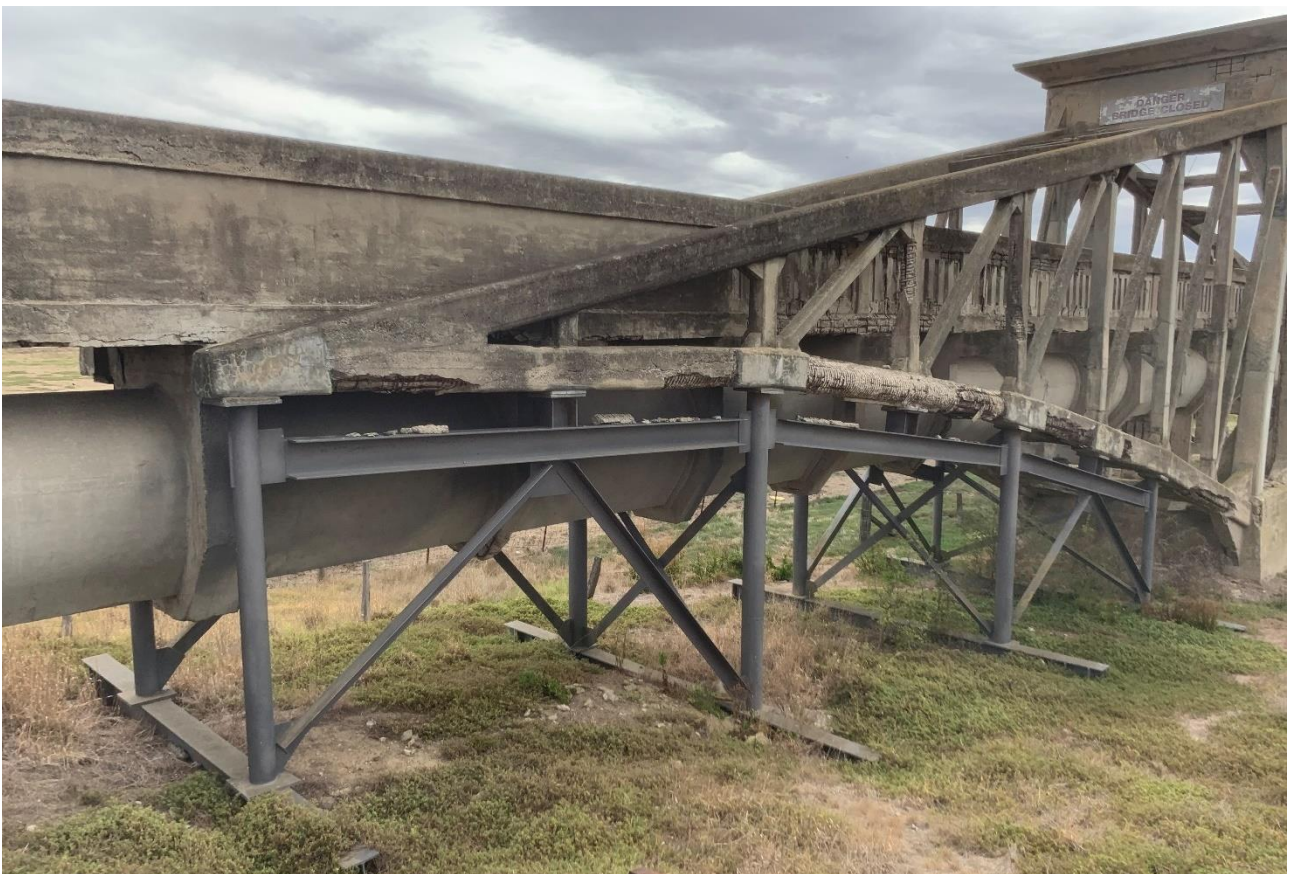
Figure 22 Steel propping installed below Truss #14 at South Landing, c. 1992 Source: Lovell Chen archives
