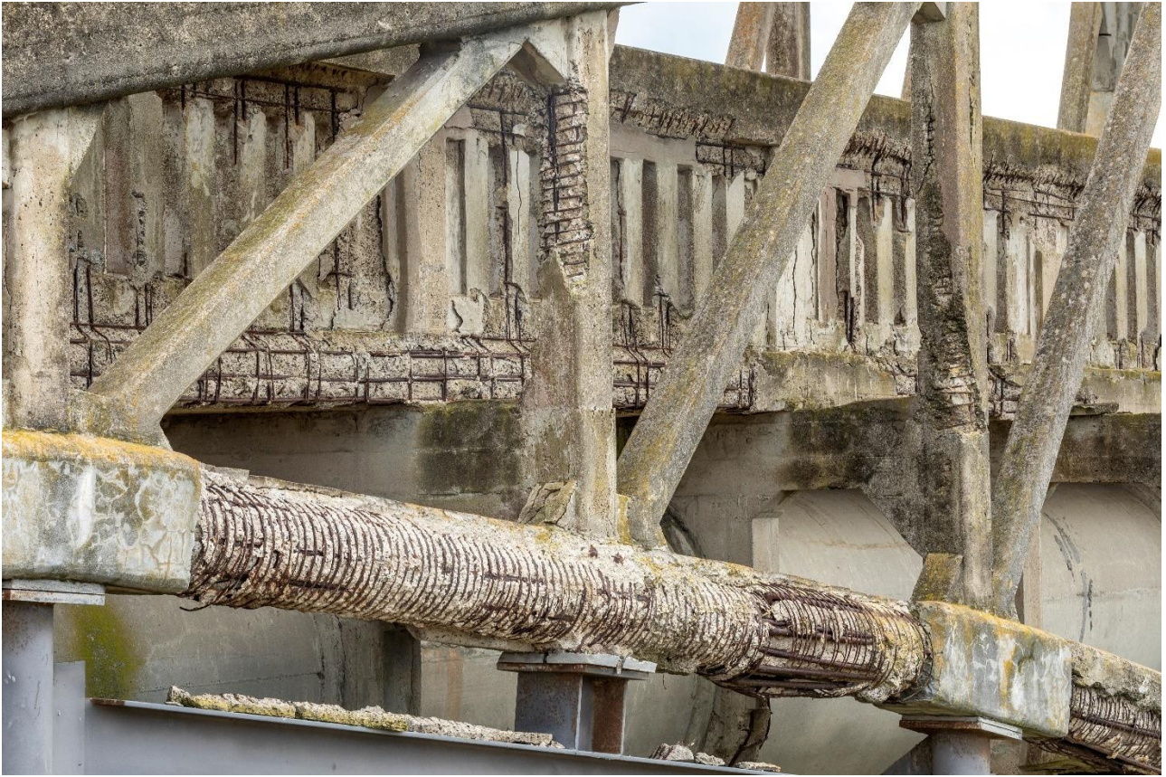
Figure 6 Extensive loss of concrete cover and exposure of steel reinforcement at Truss 14 (South Landing Site) Source: Glasshouse Creative Media, courtesy Barwon Water
