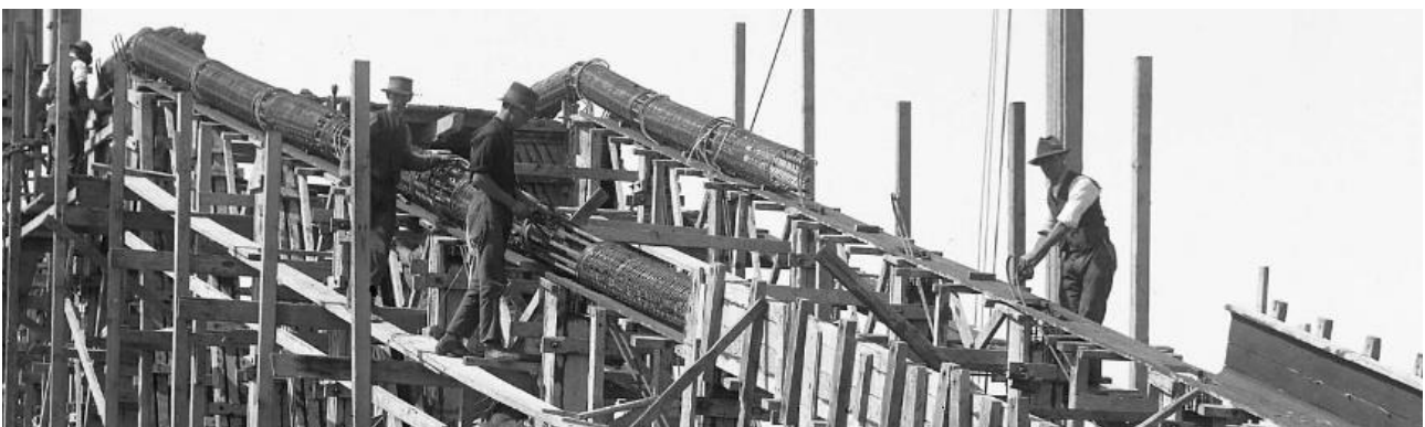
Figure 14 Detail, assembly of steel reinforcement and timber formwork for upper chord of truss (c. 1914-1915) Source: Barwon Water archives
