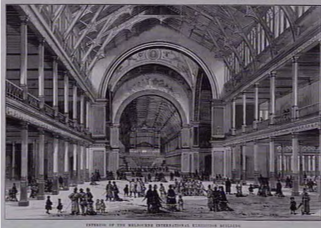
Figure 7 Interior of the Melbourne International Exhibition Building, 1880. Source: Picture Collection, State Library of Victoria.
