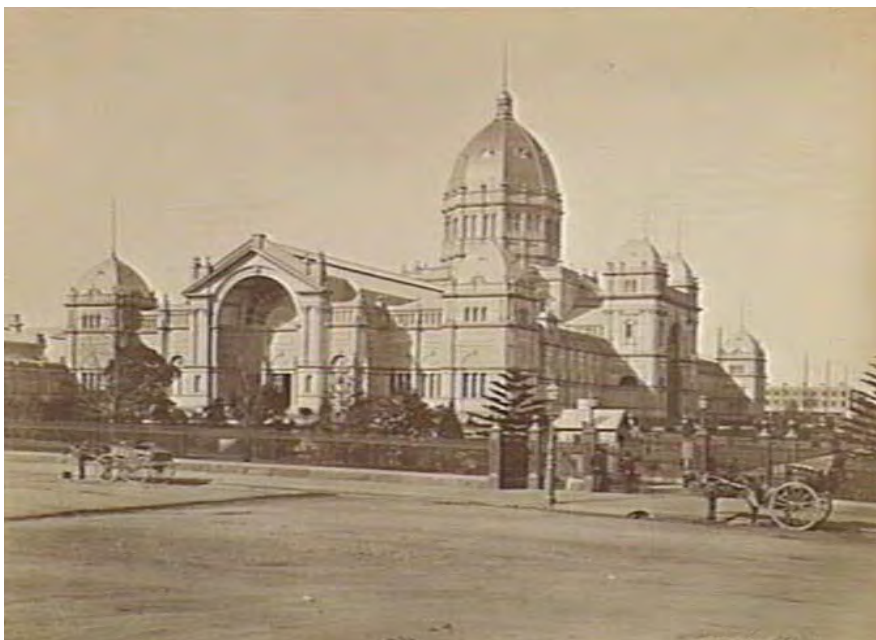
Figure 10 The Exhibition Building's western and southern elevations, with iron palisade garden fence and corner gateway (foreground) supported by decorative hollow cast pillars surmounted by finials, c. 1880.
