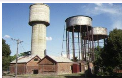
Benalla Water Supply Depot Benalla Water Tower Preservation Group Inc Benalla
