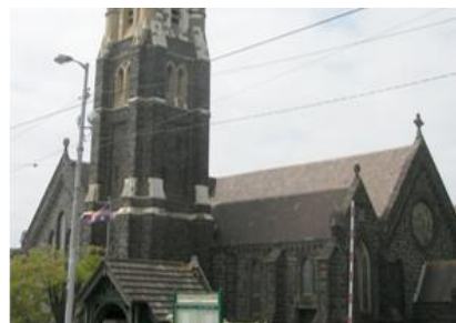
Christ Church, South Yarra Christ Church South Yarra (Melbourne Anglican Trust Corporation) South Yarra
