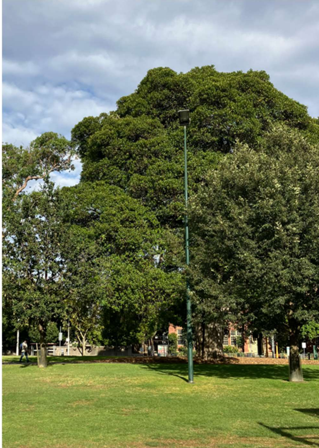
Figure 03. Existing floodlight adjacent playground on 10m pole.
