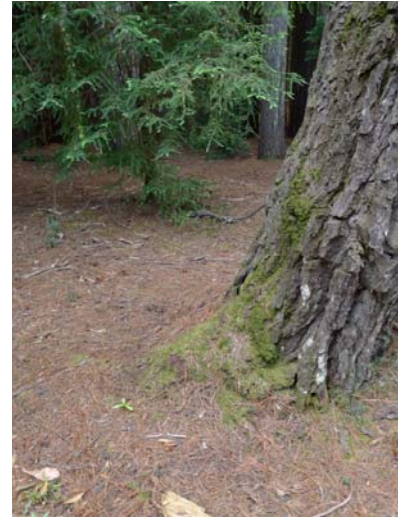
Photo 210: Tree 237 base of tree showing root heave
