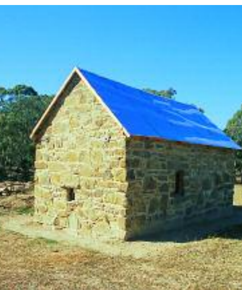
Above: Restored Stone Cottage, Barkers Creek.
