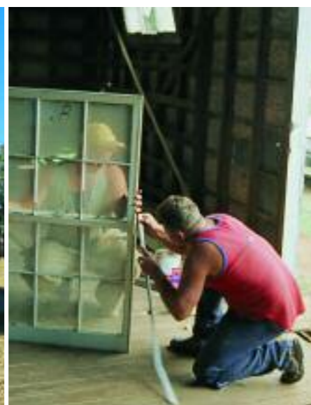
Above: Restoration at Ercildoune Woolshed.
