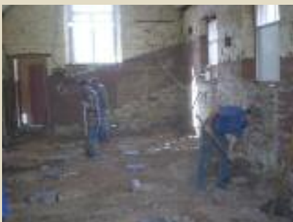
Below: Volunteers at work at Clydesdale Community Hall. The refurbished hall.
