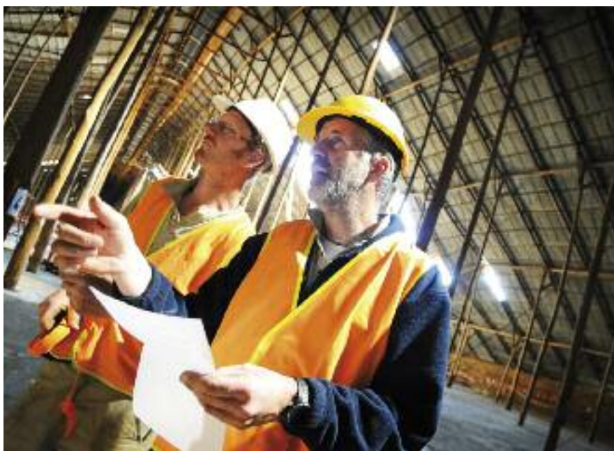
Pic: Greg Owen and Jim Mellor of Period Restoration Services, specialist building conservation contractors, discuss works to the Stick Shed.
