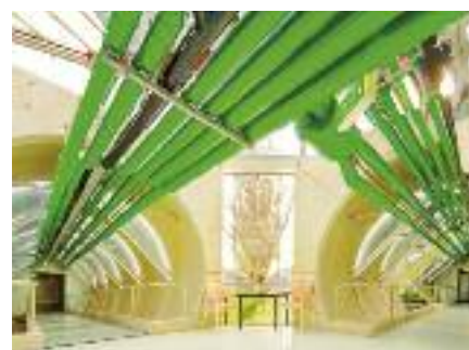
The distinctive pipe walkways at the former Clyde Cameron College. Images courtesy Murray Valley Private Hospital.
