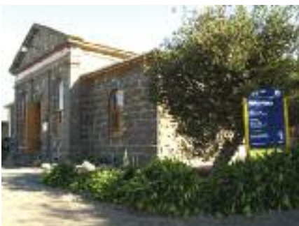
Extensive works are underway at the 1888 Portland Drill Hall, part-funded by $100,000 Heritage Grant, to replace flooring, external weatherboards, restoration of ceiling, internal truss roofing, etc. It had been in a very dilapidated condition.
