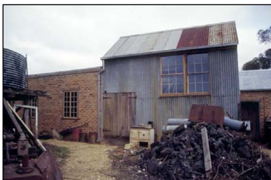
Battery Shed (after repair)
