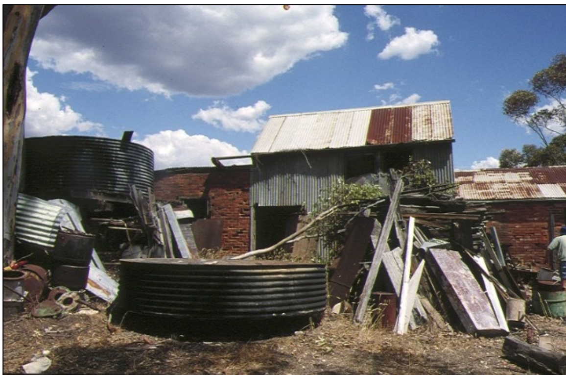
Battery Shed (prior to repair)
