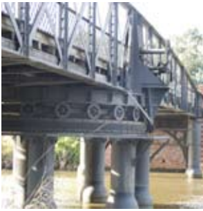
The Swing Bridge at Longford (H1438) near Sale has been restored and is regularly swung open.
