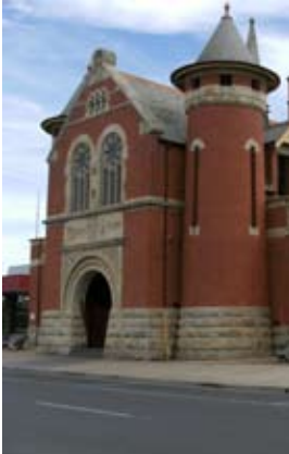
Bairnsdale Court House Bairnsdale Court House (H1462) is in an extravagant Federation Romanesque style.
